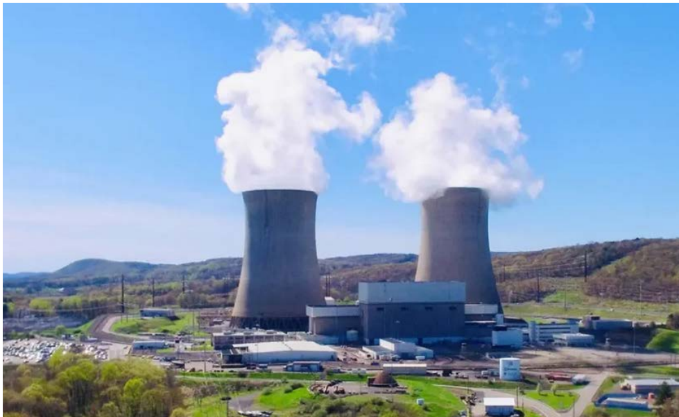
Co-location of data centers with zero-emissions energy resources such as the Susquehanna nuclear power plant was discussed during a WECC webinar. | Talen Energy
