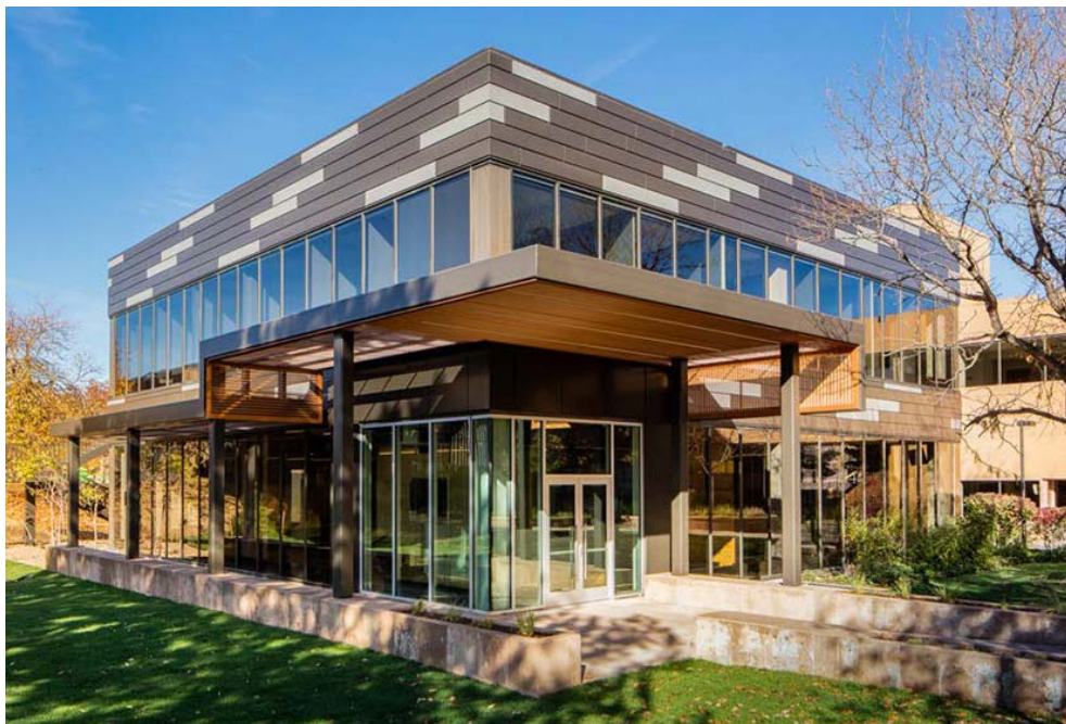
Data centers can come online as quickly as 18 months, potentially adding large loads to the grid, according to WECC. | H5 Data Centers
