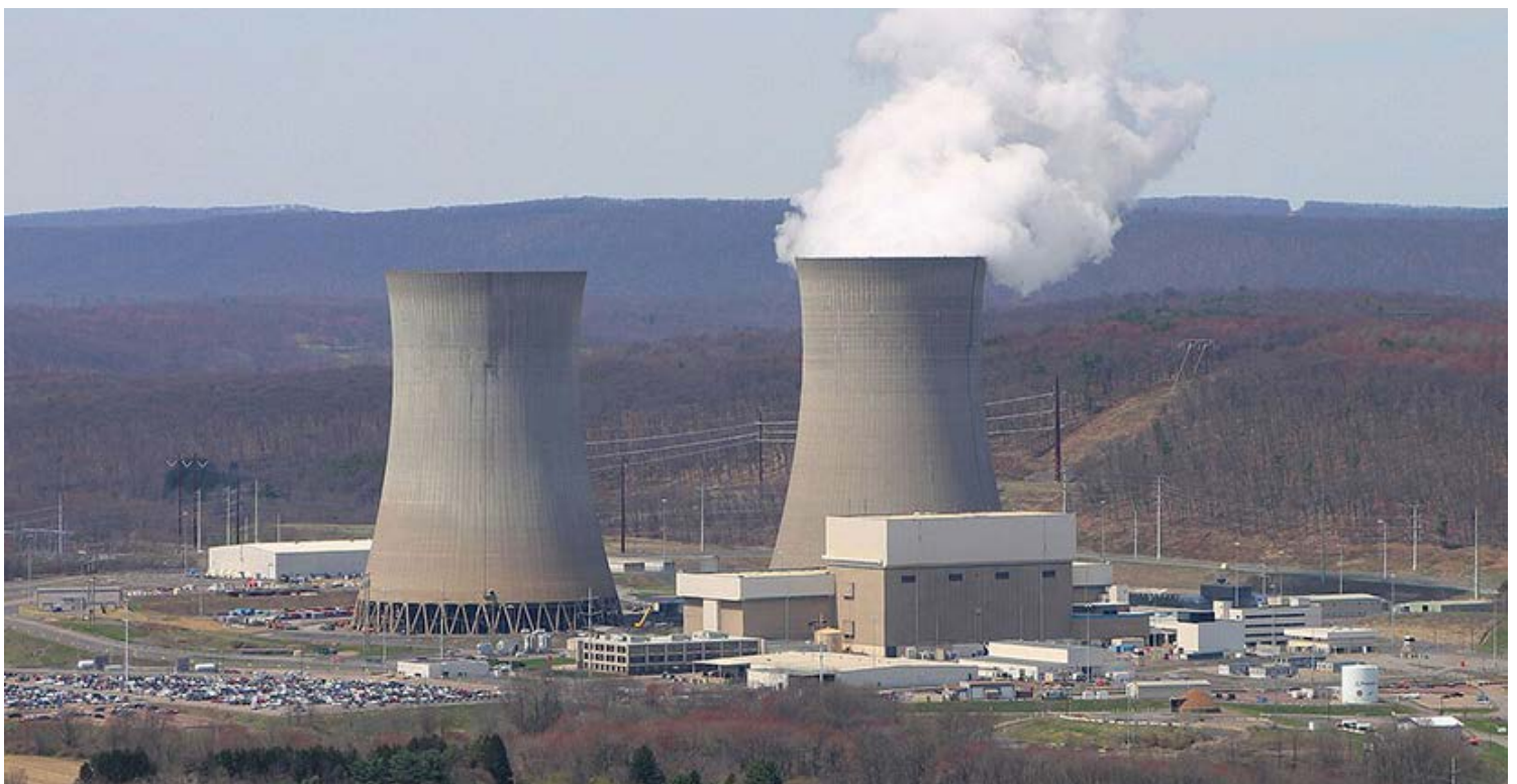
Talen Energy's Susquehanna Nuclear Power Station | Jakec , CC BY-SA 4.0, via Wikimedia Commons
